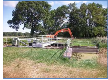
2019 Baubeginn © StALU VP
